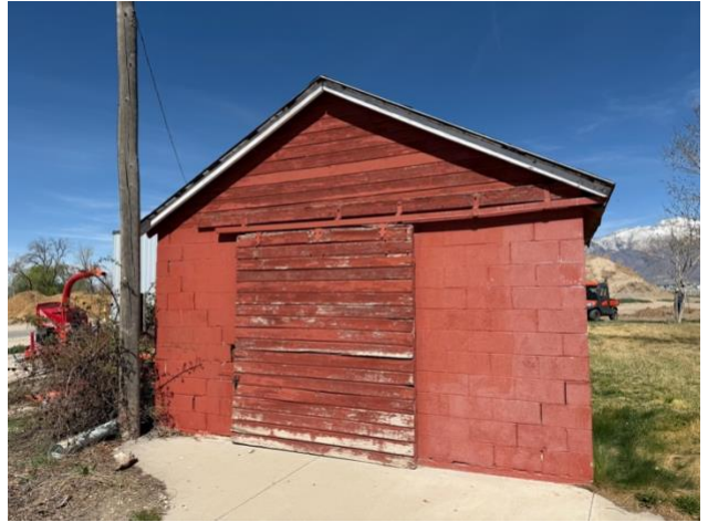
PHOTO 2: Utah State Developmental Center, Storage Shed
