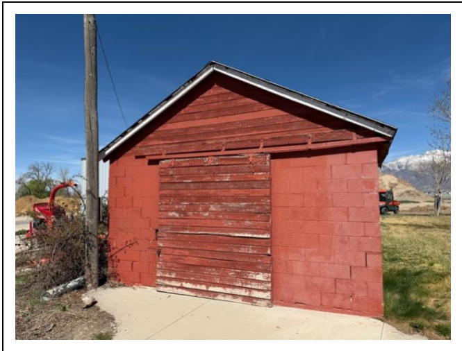
PHOTO 3: Utah State Developmental Center, Storage Shed
