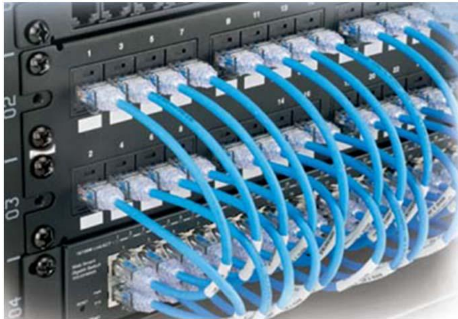
Example of one-to-one switch patching
